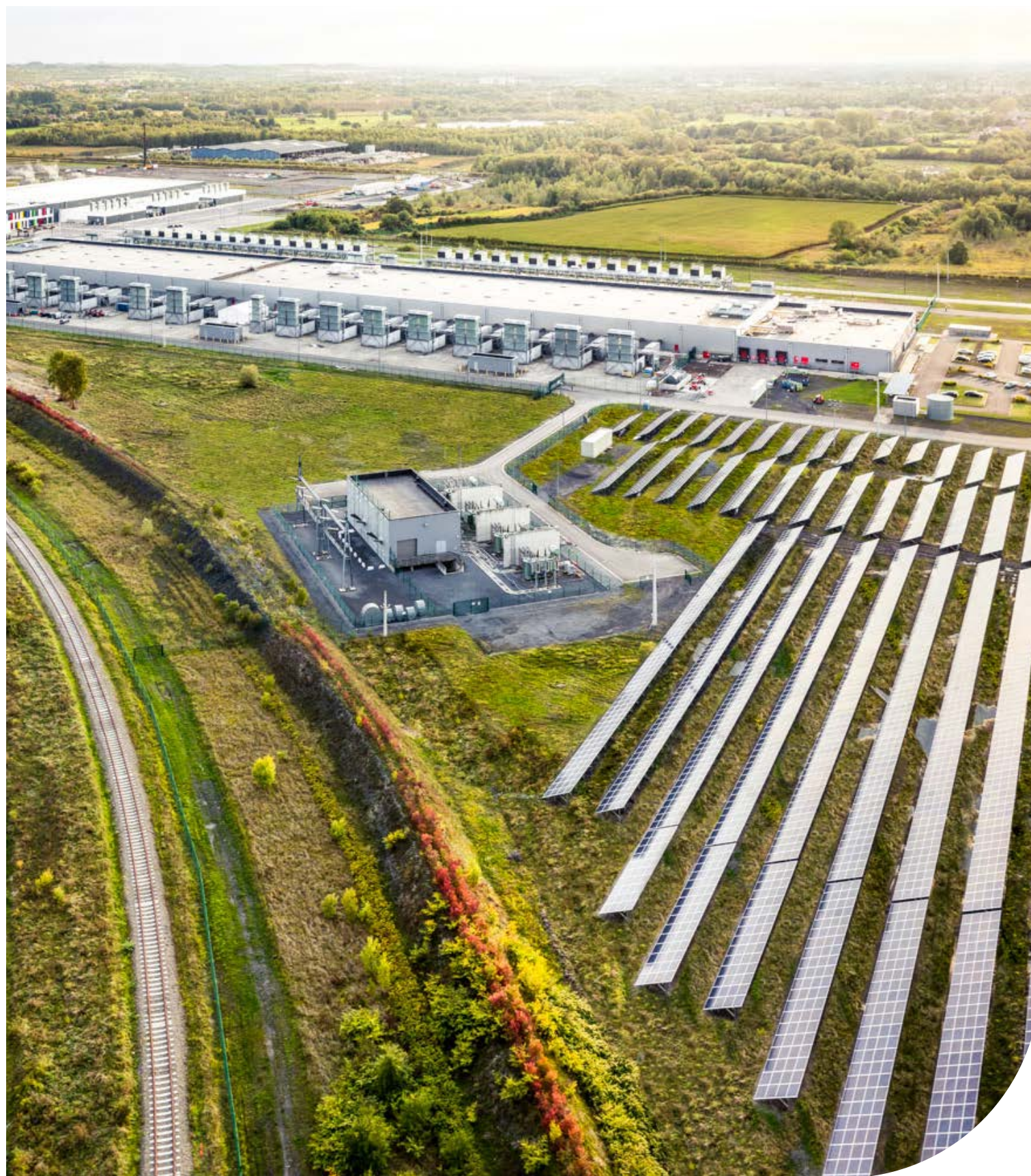
Google's data center in St. Ghislain, Belgium.
