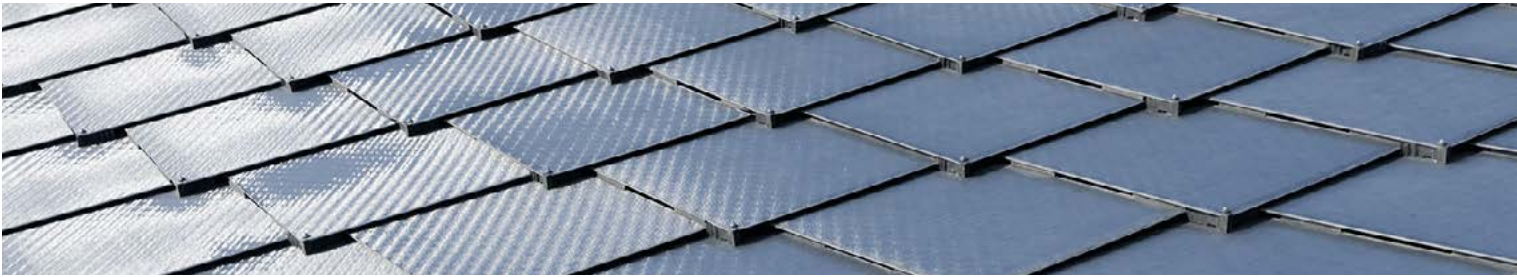
For our Bay View campus, a first-of-its-kind building-integrated solar panel called “ dragonscale ” was developed to create a seamless design. (Photo: Iwan Baan)
