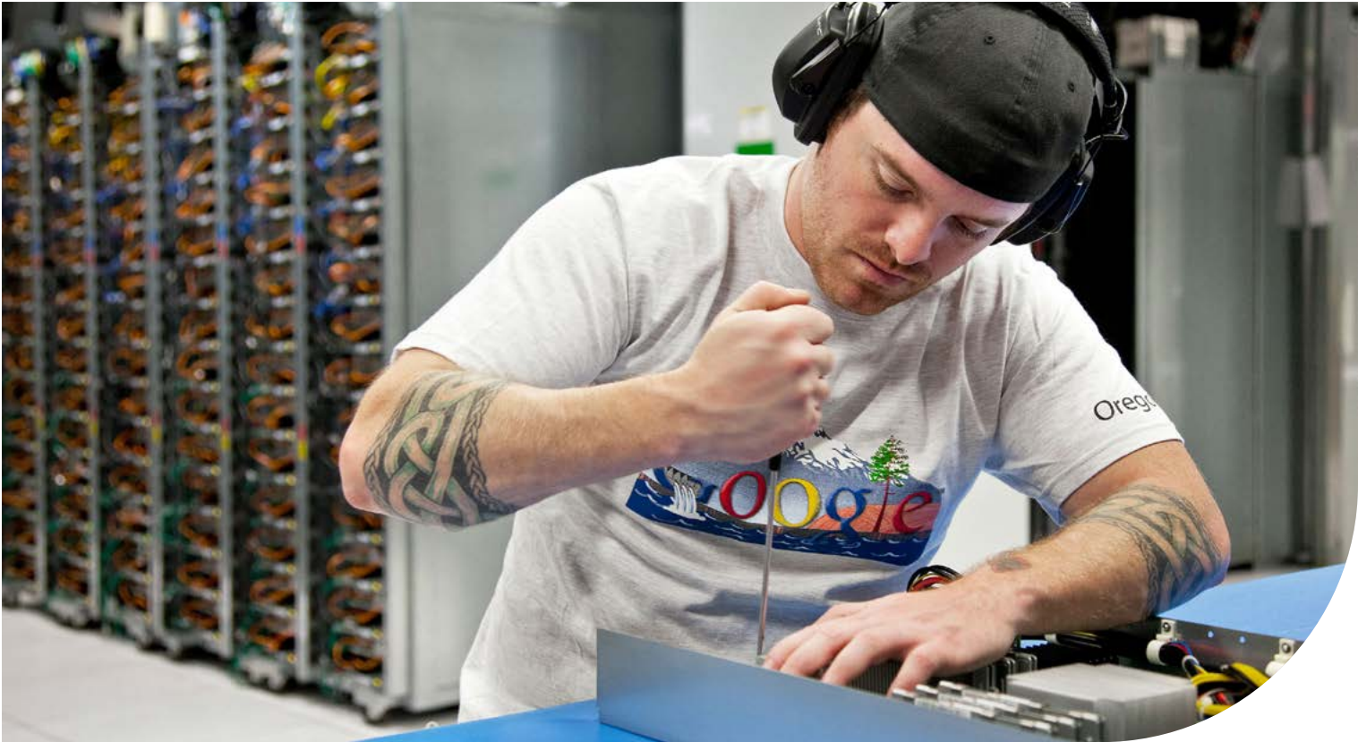
A Googler swaps out a motherboard at our data center in The Dalles, Oregon. When server parts break, we first try to repair them. If we can't, we break them up into raw materials and recycle the components.
